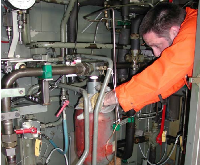
Fig. 1 Maintenance technician during maintenance work
