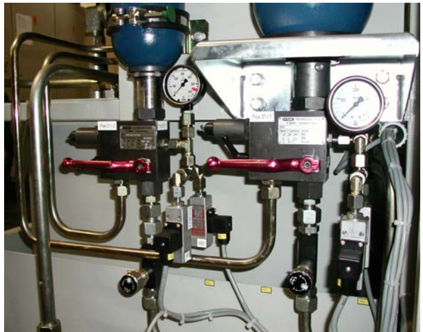
Fig. 25 Depressurized hydraulic accumulators with closed pressure lines
